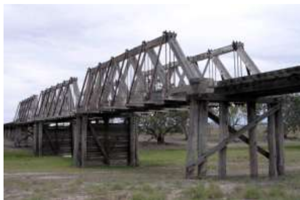
Plate 6 – Two Mile Warrambool railway bridge.
