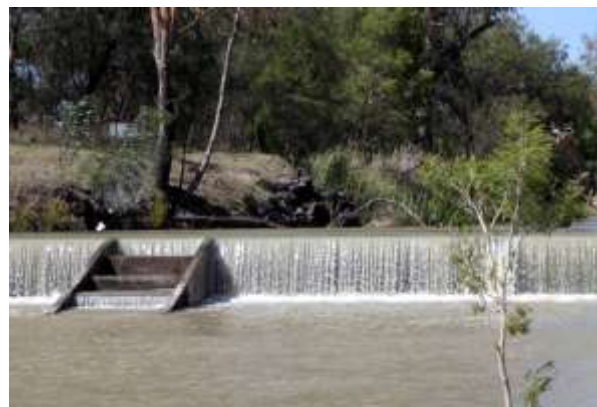
Plate 6 – Fish ladder on the Collarenebri weir.
