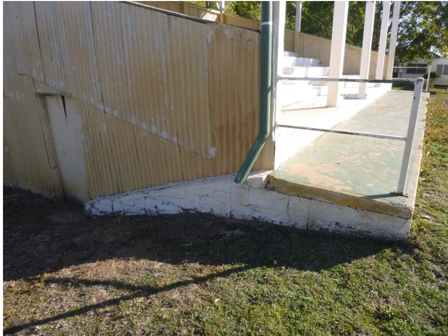
Figure 11 – Downpipes discharge to ground on the east and west elevations.
