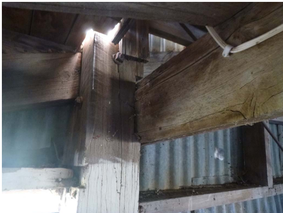
Figure 16 – Failure of the timber support beam at the timber column.
