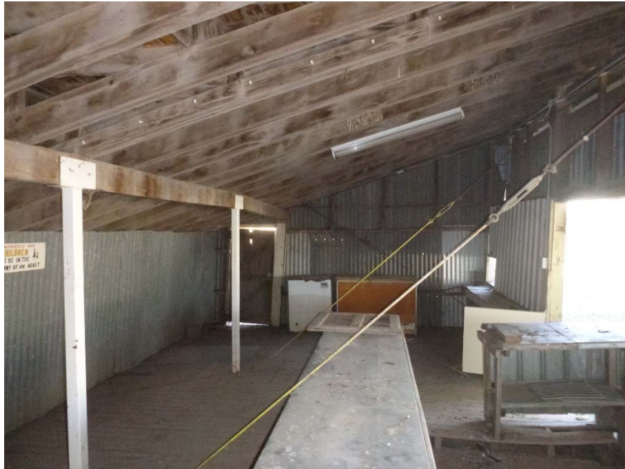
Figure 17 – The grandstand external wall has settled relative to the steel columns.
