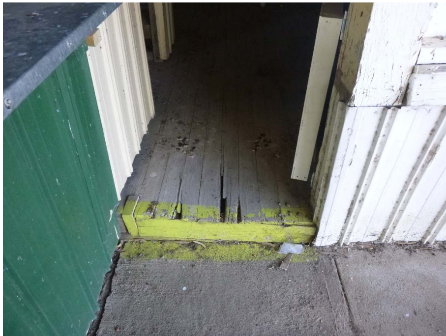
Figure 19 – Deterioration of timber floor boards.
