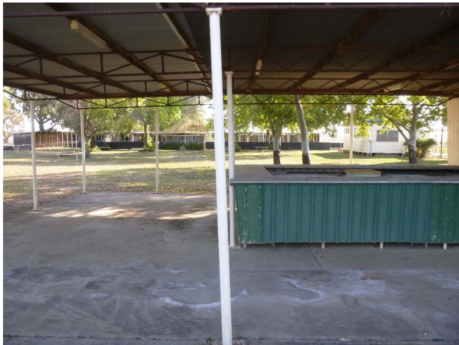
Figure 25 – Columns are no longer vertical.
