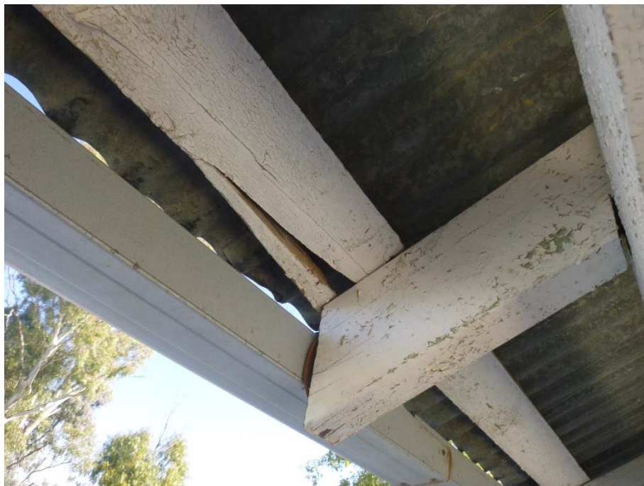
Figure 8 – Timber batten split.
