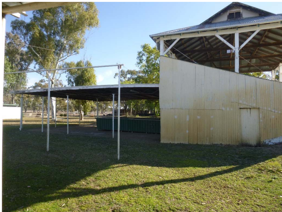
Figure 12 – The southern wall of the grandstand has settled and rotated to the south.
