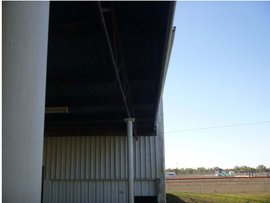
Figure 24 – Eastern lightweight steel truss has started to buckle.
