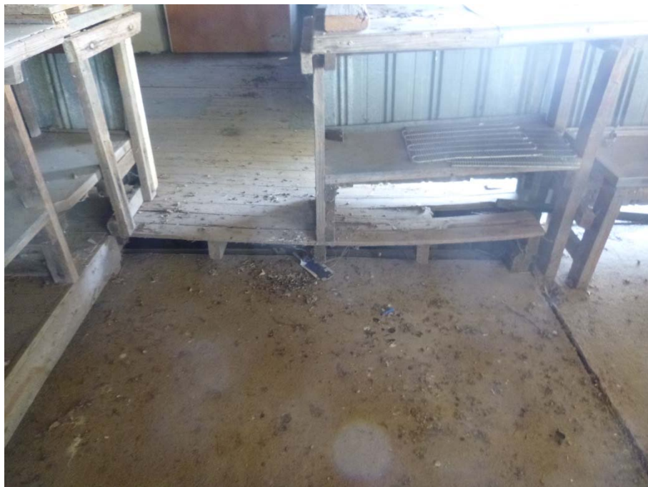
Figure 20 - Deflection of timber flooring.
