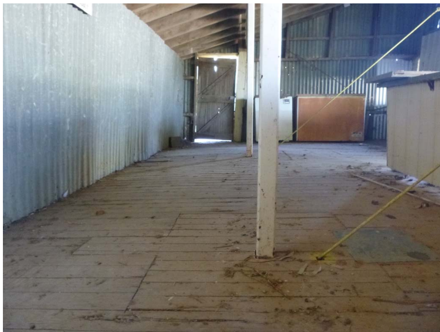
Figure 18 – Timber flooring is very uneven.
