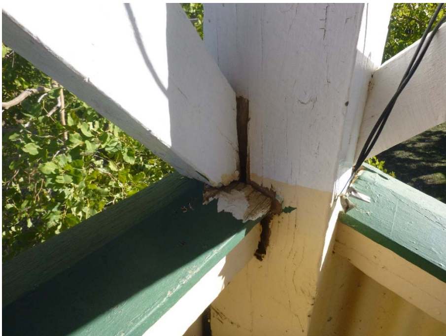
Figure 10 – Various timber connections are compromised.
