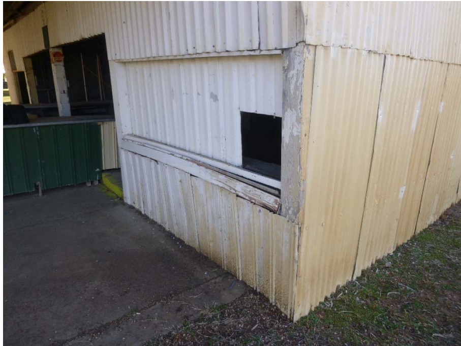
Figure 21 – Settlement of the southern wall has caused the timber framing to buckle.
