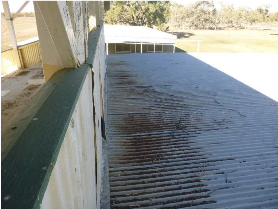
Figure 9 – External cladding is damaged throughout.
