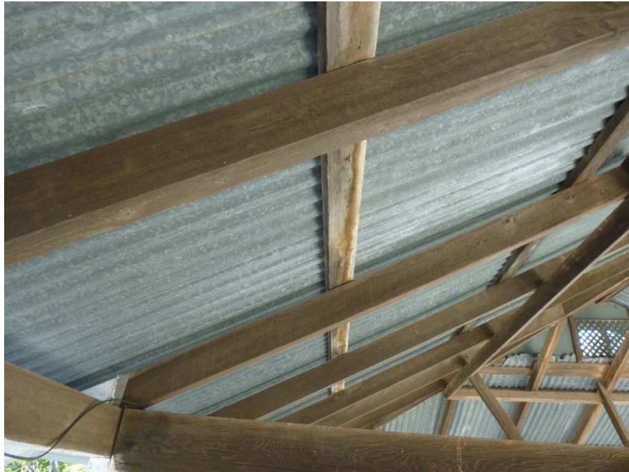
Figure 7 – Moisture staining to various timber battens.
