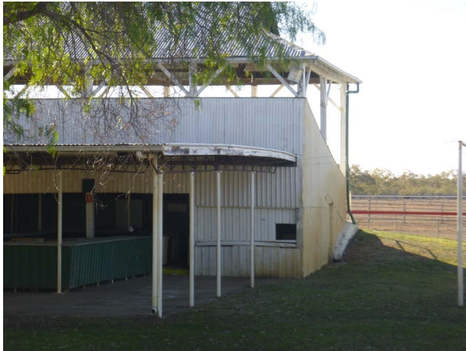
Figure 22 – The roof is not straight and is back falling to the building.
