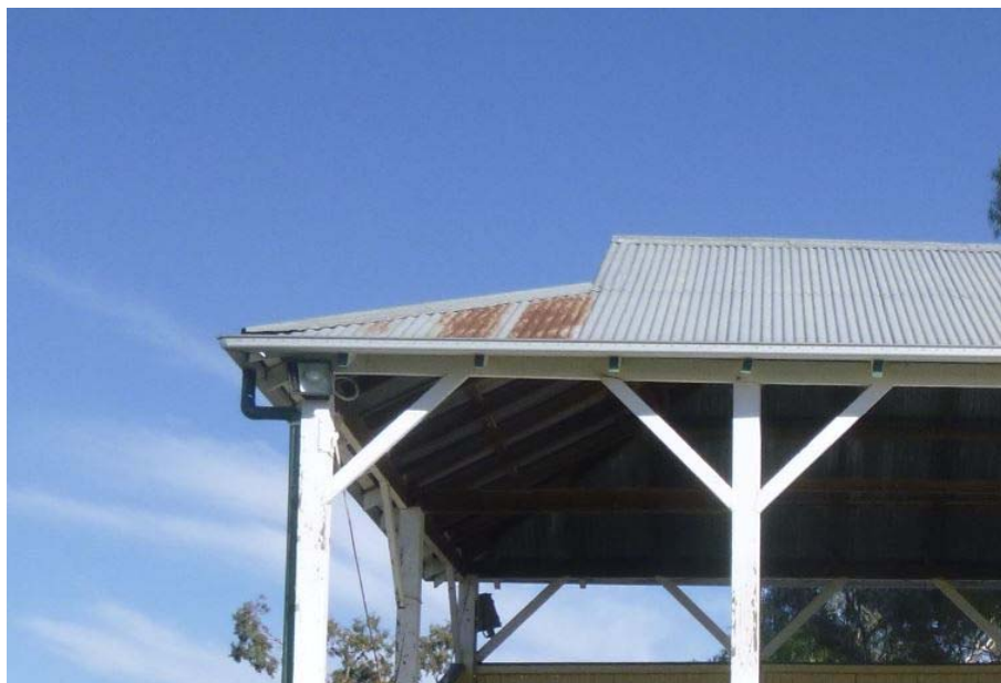
Figure 13 – The roof sheeting has reached the end of its design life.
