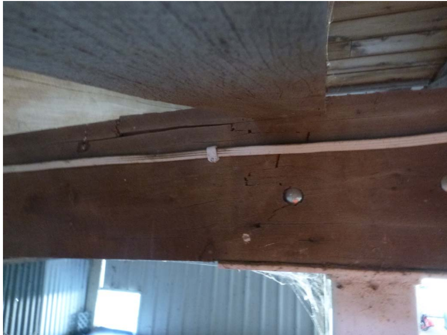
Figure 15 – Splitting to the bearer beam over the steel column.
