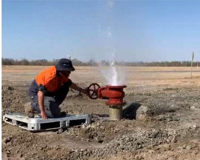
Council is planning to install new six flush points on various streets in Collarenebri. Attached is one of the new flush points that was installed in George Street.
