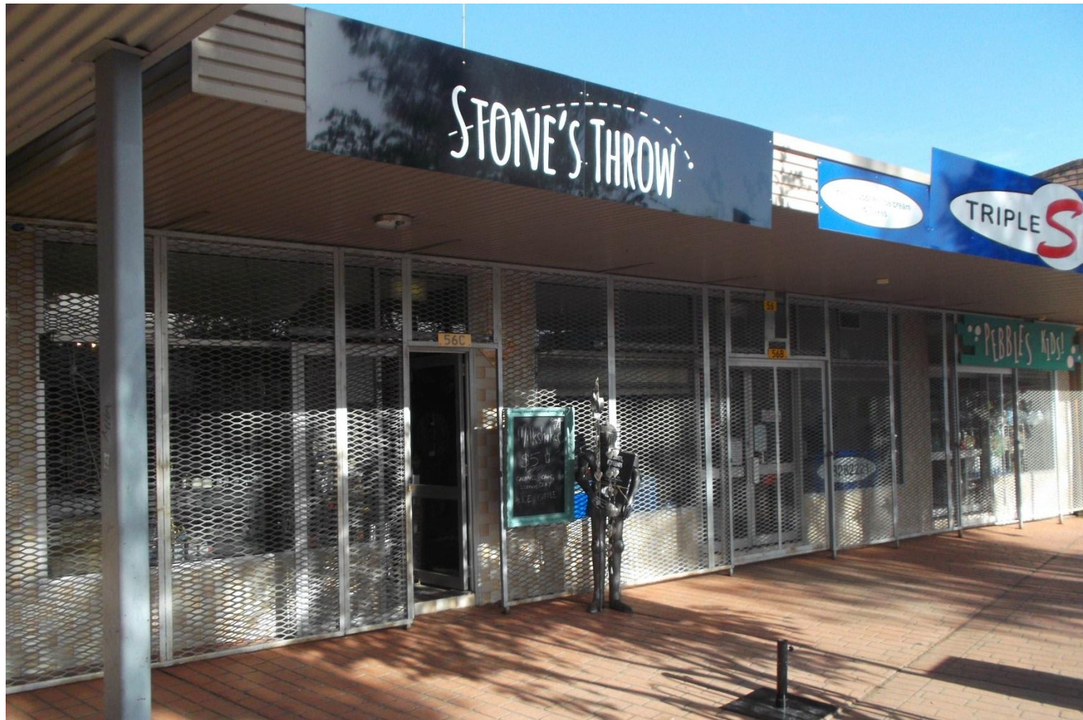
ATTACHMENT B – 16-12-2014 photograph of existing expanded mesh security screen
