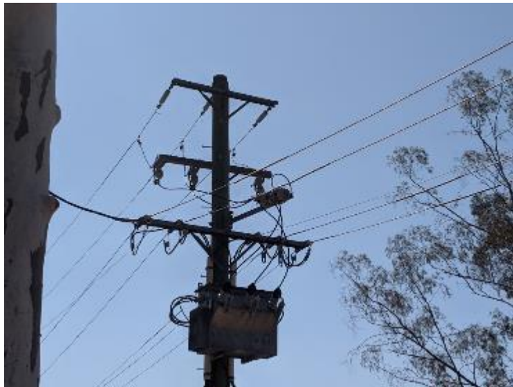
Figure 12-1: Existing transformer serving the Lighting Ridge depot and reservoirs
