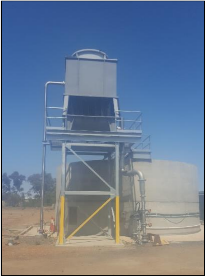
Figure 1: Walgett Water Supply Cooling Tower & Balance Tank.
