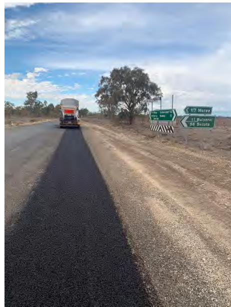
Photo during Pot hole repair and spray seal on Merrywinebone Road
