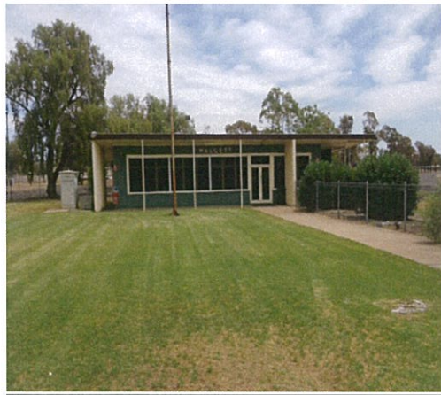
Walgett Airport Terminal
